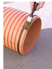
Mazanje PVC rebraste cevi in tesnila
