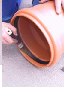
. . . ter PVC cevi in tesnila
